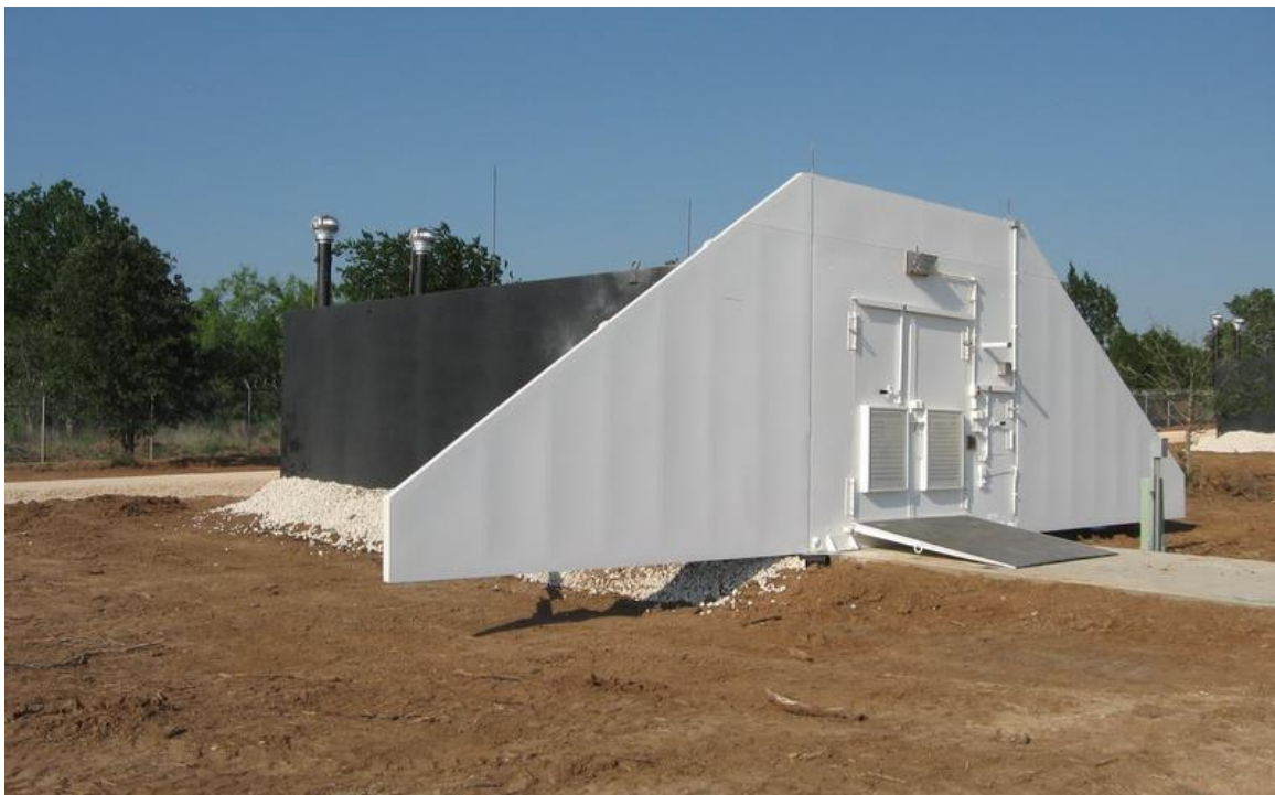
Figure 1 - An Armag 3-Bar ECM during installation. The fold-out steel retaining walls facilitate quick and easy installation.
